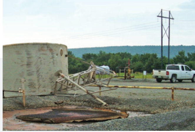
A Chesapeake tank is damaged after being struck by lightning prior to the installation of grounding technology.
